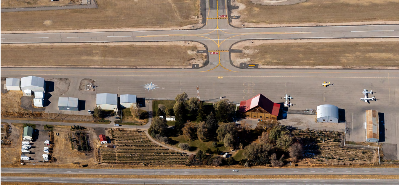
Figure 4.21: East General Aviation Apron
