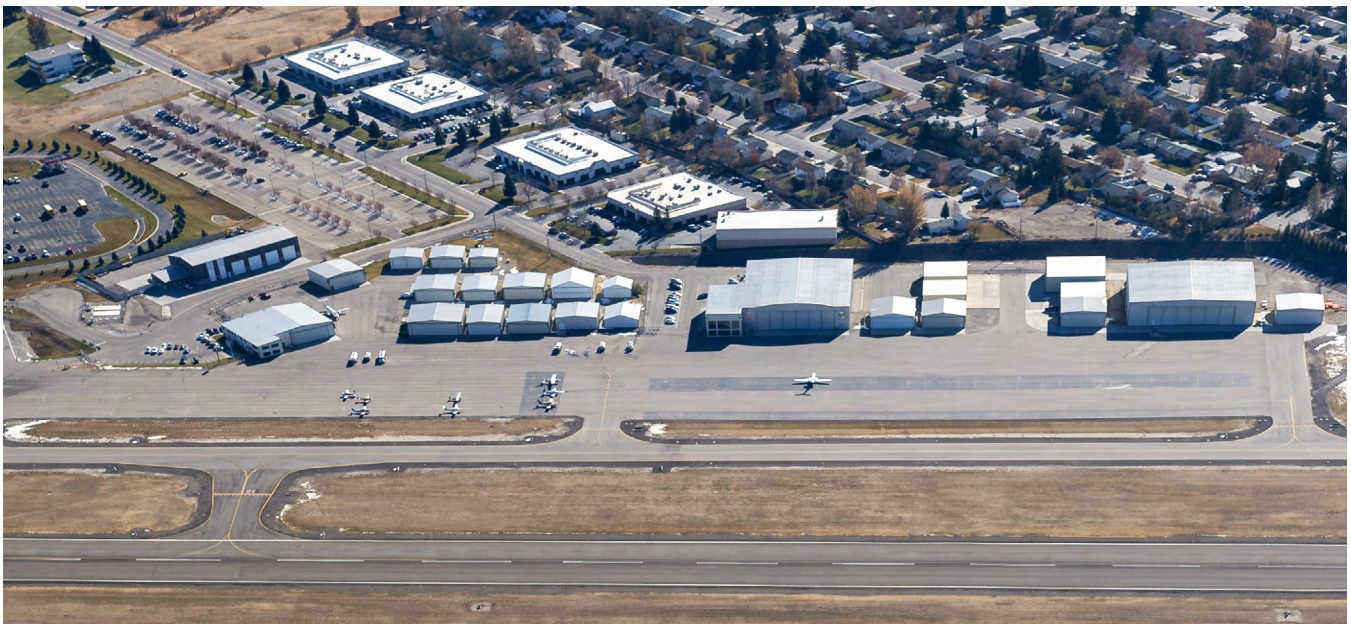
Figure 4.20: Main FBO Apron
