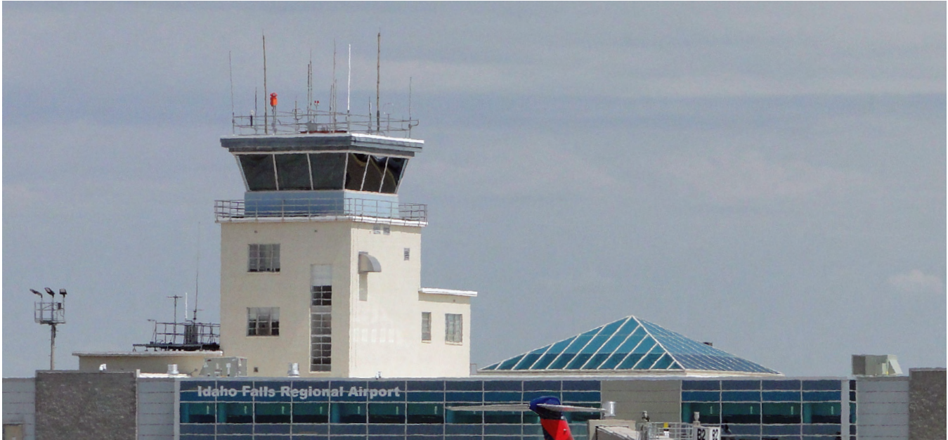
Figure 4.24: Airport Traffic Control Tower
