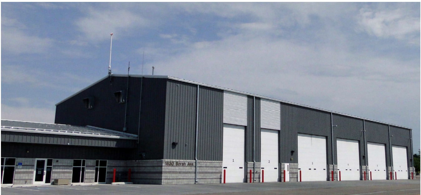
Figure 4.30: Snow Removal Equipment Facility
