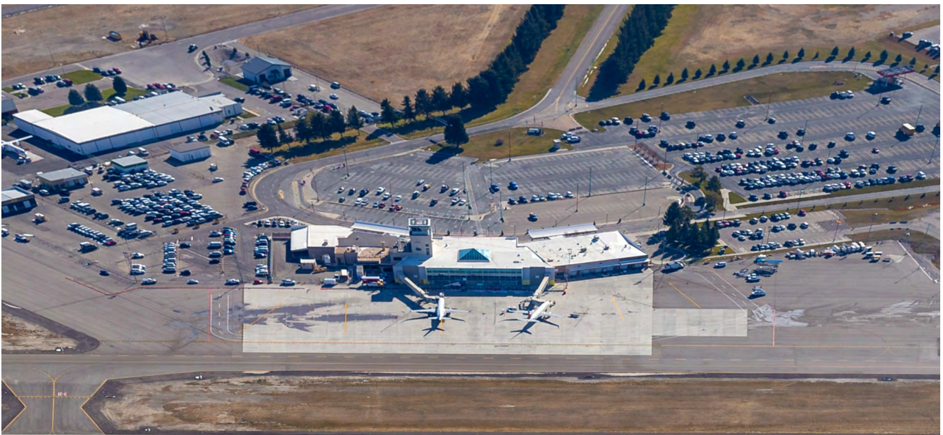
Figure 4.22: Commercial Terminal Apron
